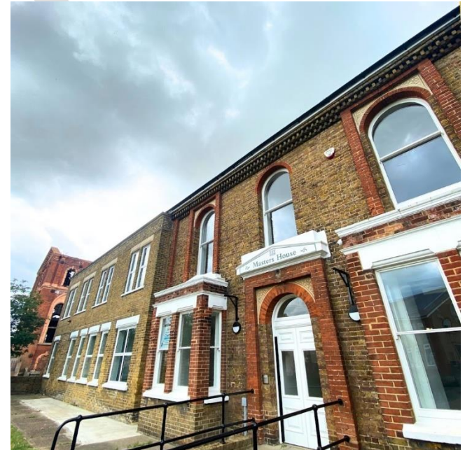
A refurbished Master's House, Sheerness.
