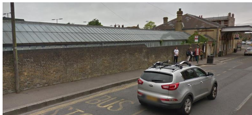
Existing boundary wall along the southern side of Station Road.
