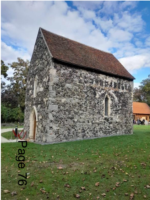
The recently restored Murston Old Church where the Green Grid was hosted.
