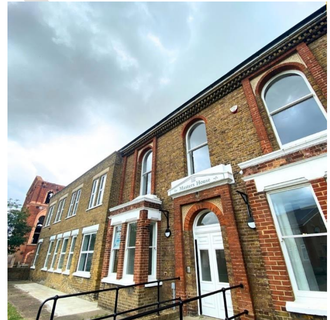
A refurbished Master's House, Sheerness.
