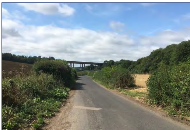
View south along valley bottom at Bottom Pond Road, showing M2 on viaduct
