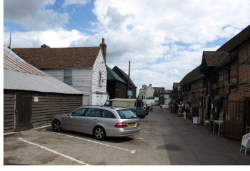
Standard Quay cluster of listed buildings and an important part of the association with the creek.
