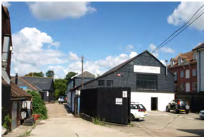
The Swan Quay site 5 with the listed chandlery building which should be retained.
