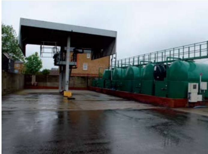
Storage buildings and retaining wall
