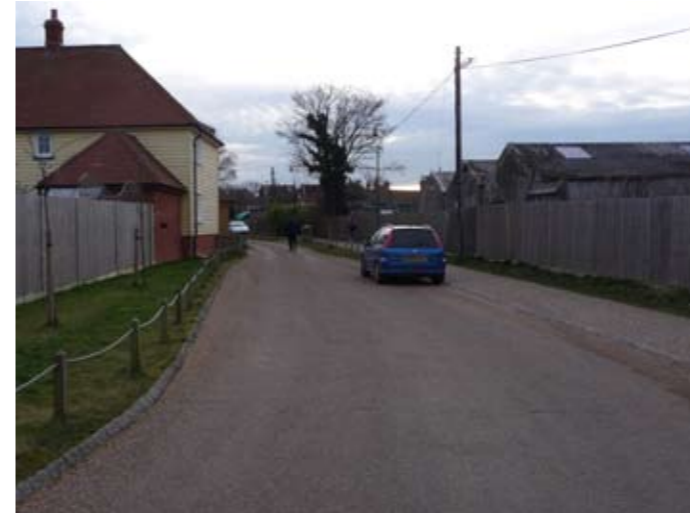
Rear boundary wall to the New Creek Road
