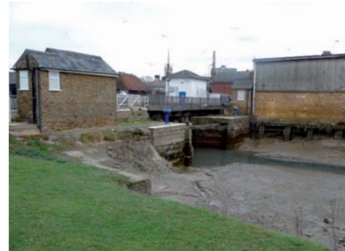
The bridge and sluice at the entrance to the creek basin
