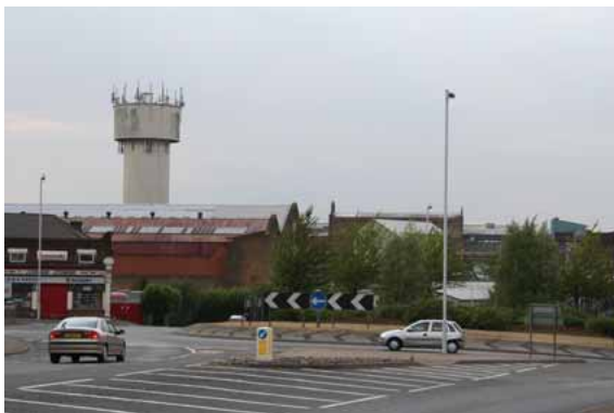
View towards the Paper Mill
