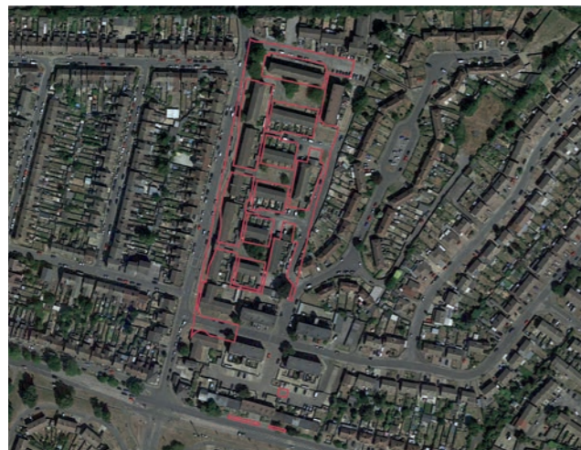
Site 140 aerial view
