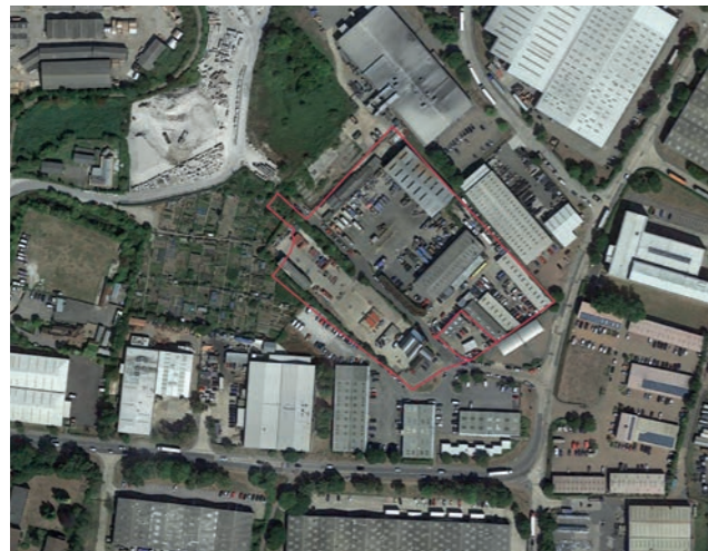
Site 95 & 102 aerial view
