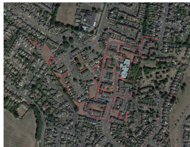
Site 121 & 159 aerial view
