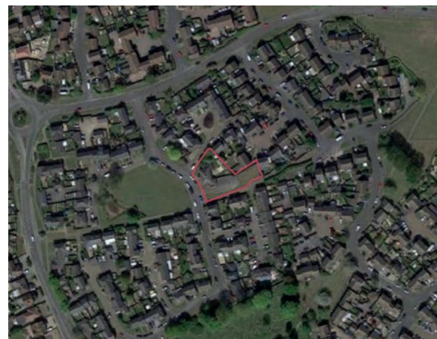
Site 1 aerial view
