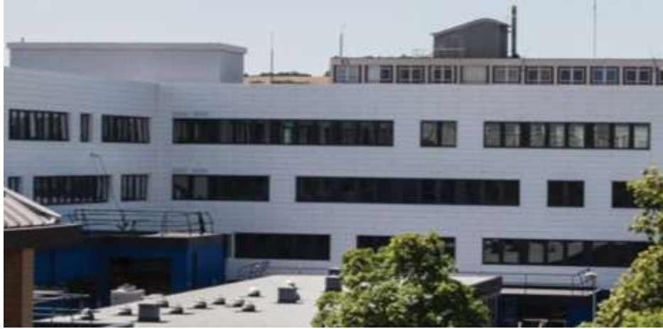
Figure 12: Before and after photos of cladding installation at RAL site, Didcot, Oxfordshire.
